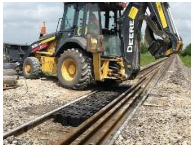
There's no need to have local law enforcement on hand to redirect traffic or close crossings for repairs. From start to finish, Turtle Trax installs in less than two minutes, using either sledge or air hammer. Puzzle design locks the multiple pieces securely in place.
